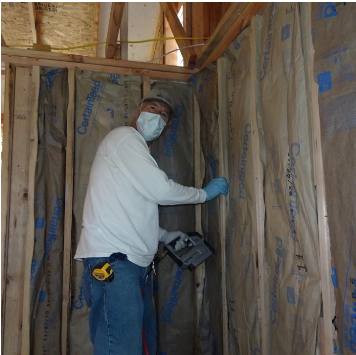
Service Project - Installing insulation in new cottages for Casa de Abuelos
